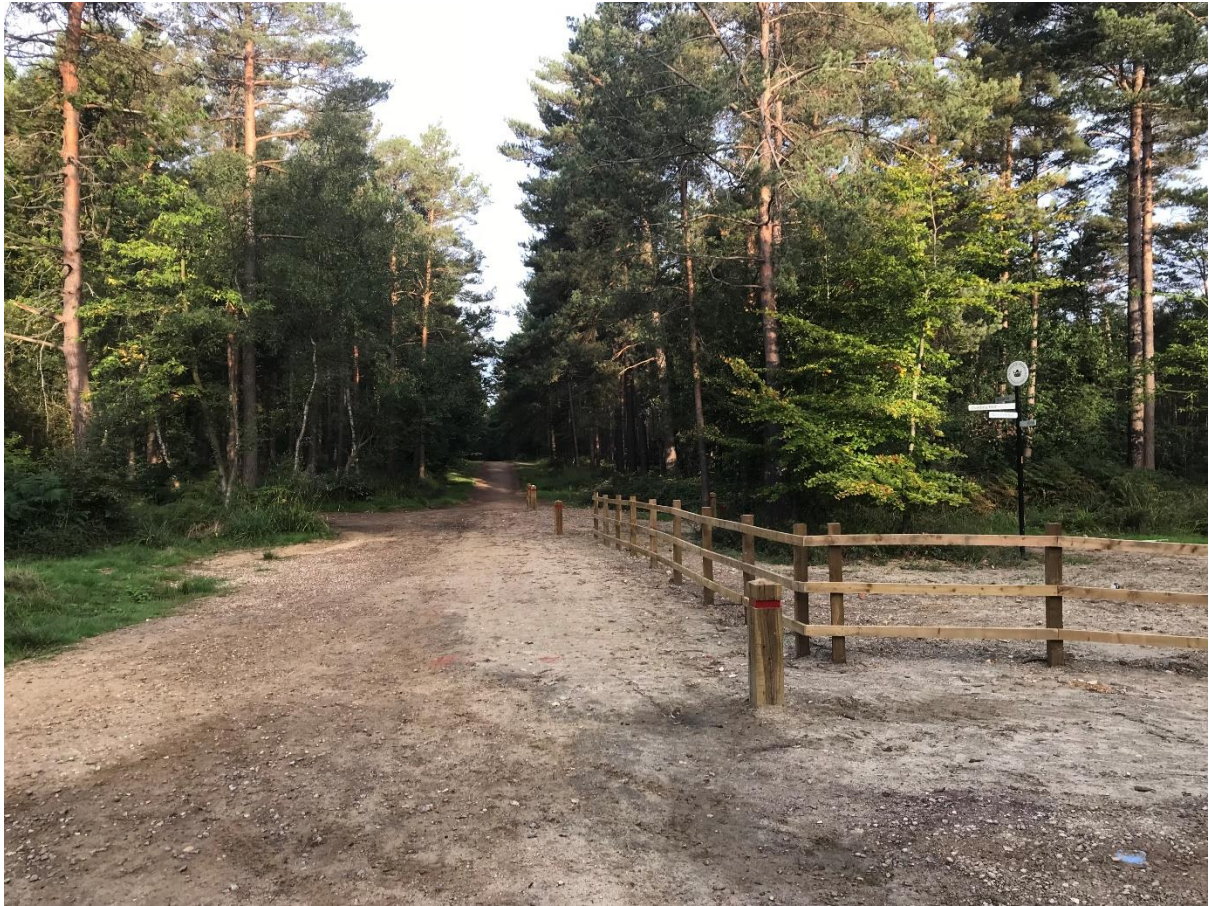
Final Junction at the end of Bracknell Road
